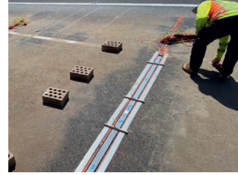
Installing the Kistler Lineas sensors – the centerpiece of the new KiTraffic Plus Weigh In Motion system on the A6 motorway in Luxembourg
