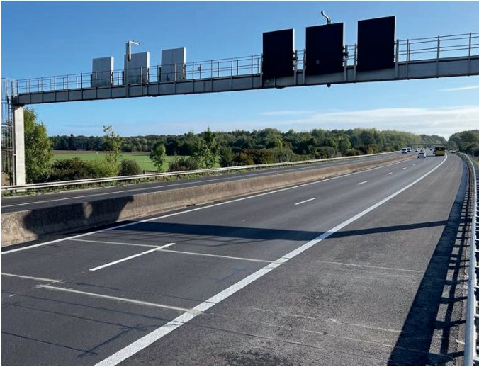
Lineas sensors installed on the A6 in Luxembourg for Weigh In Motion and more, with KiTraffic Plus by Kistler: it was possible to use the existing sign gantry for the camera systems.
