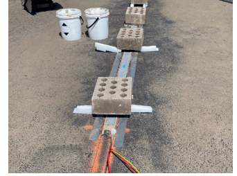
Installing the Kistler Lineas sensors – the centerpiece of the new KiTraffic Plus Weigh In Motion system on the A6 motorway in Luxembourg
