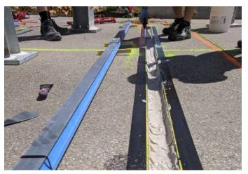
The Lineas sensors for the KiTraffic Statistics WIM system by Kistler are installed slightly below the road surface; they are coated with a special grouting compound to ensure longer lifetimes.
