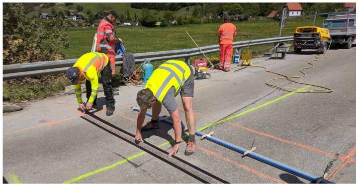
Bridge monitoring by REVOTEC on behalf of Austrian Federal Railways: installing two rows of Lineas sensors for KiTraffic Statistics.
