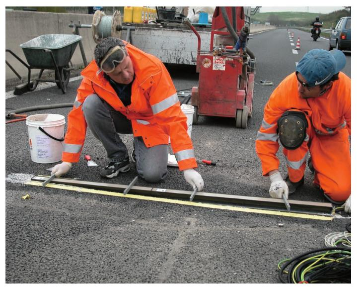
Installation of a Lineas WIM sensor.
